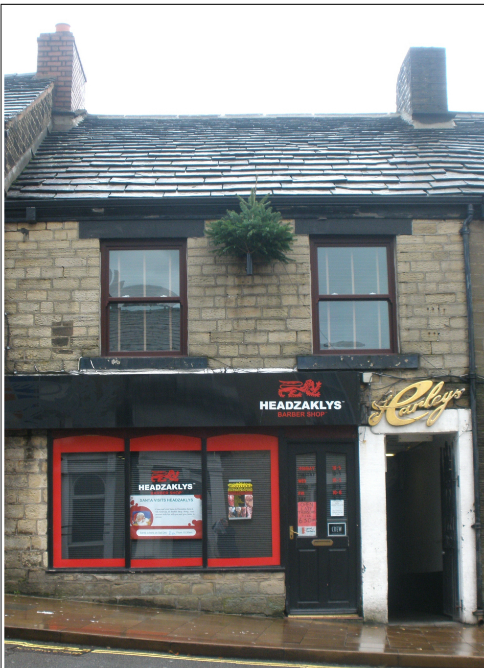
Existing Shop Front
